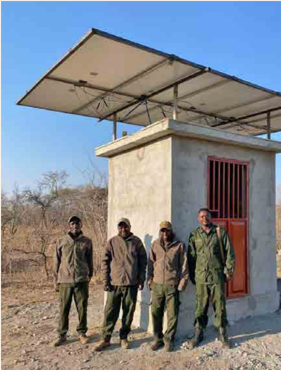
Solar panels for powering the water pump.
